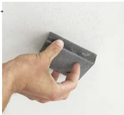
Step 03 Sanding to a finish if required
