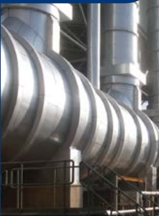
Severn Power CCGT Power Station, Uskmouth Bespoke Acoustic Barrier System
