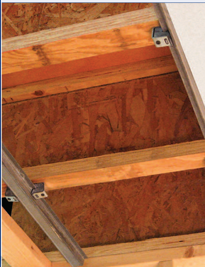
Typical construction using the IsoMax Clip to isolate walls and ceilings
